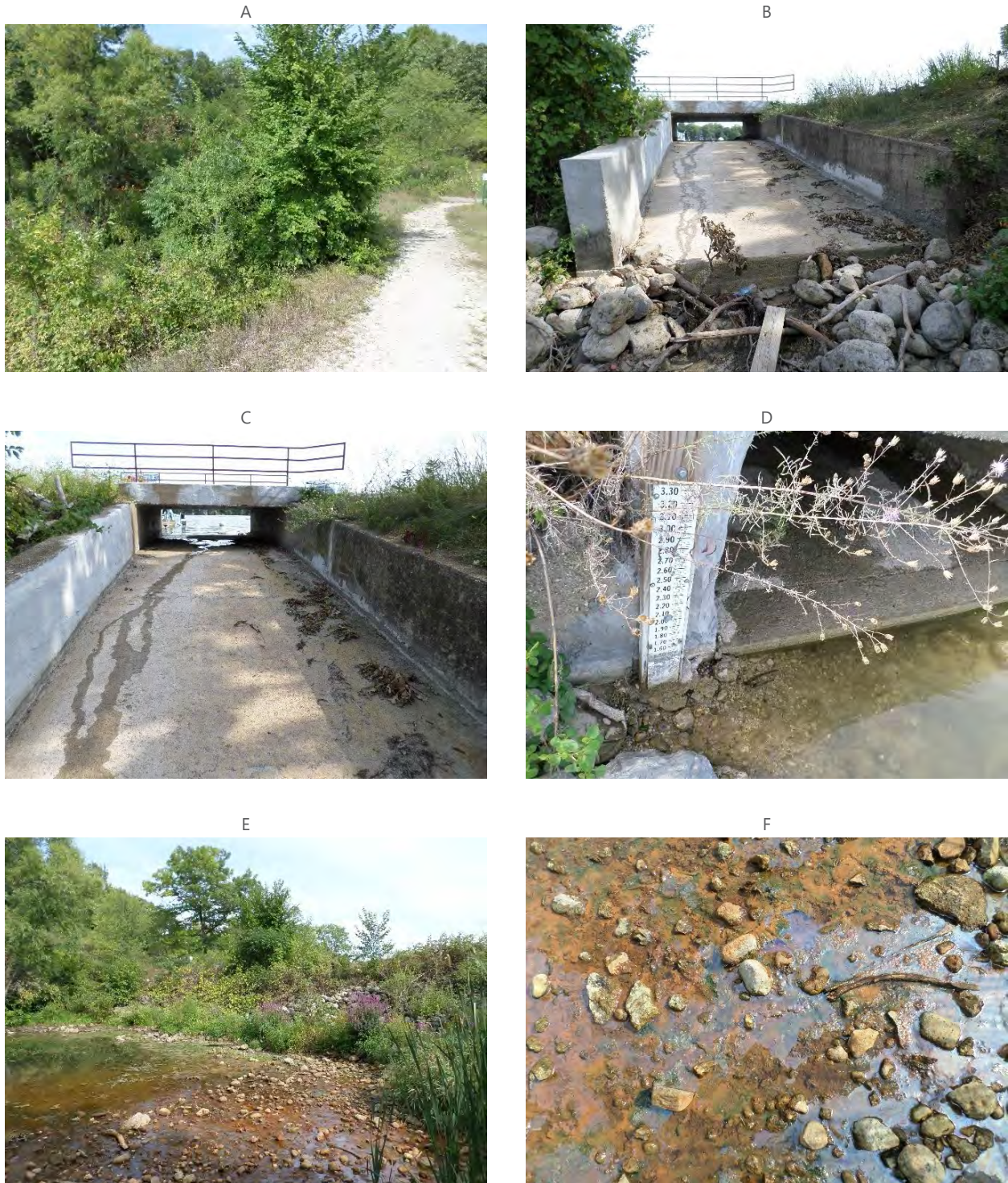
Figure 2.7 Assessment of the Whitewater Lake Dam, September 2, 2021
